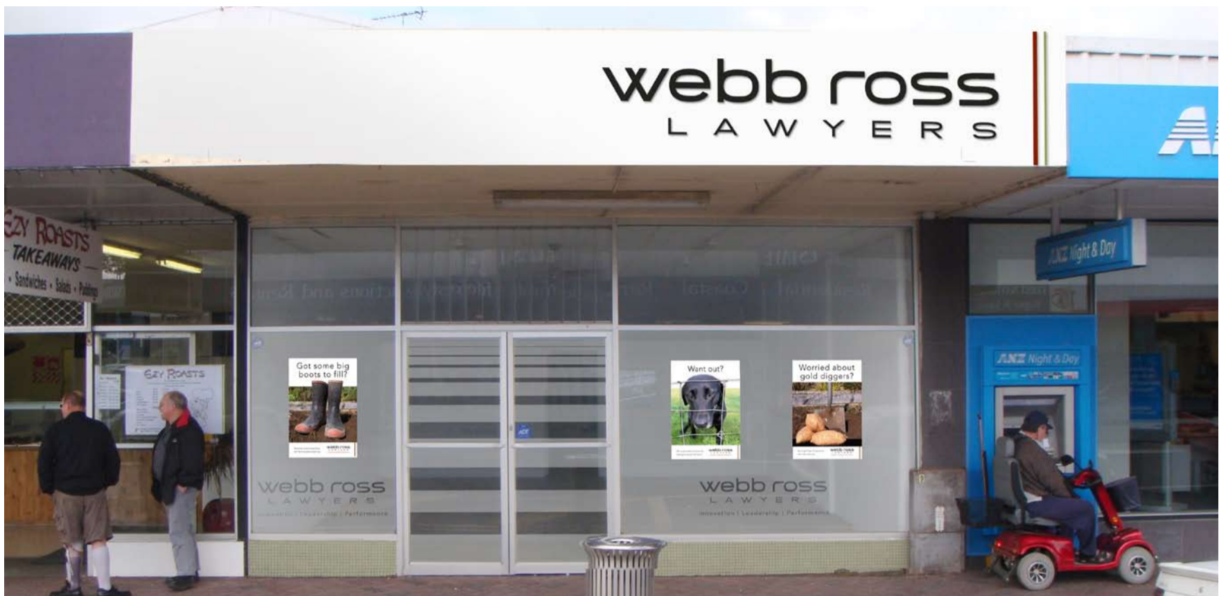
The new Webb Ross premises at 109 Victoria Street, Dargaville
