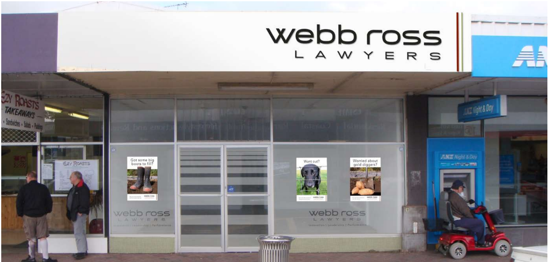
The new Webb Ross premises at 109 Victoria Street, Dargaville
